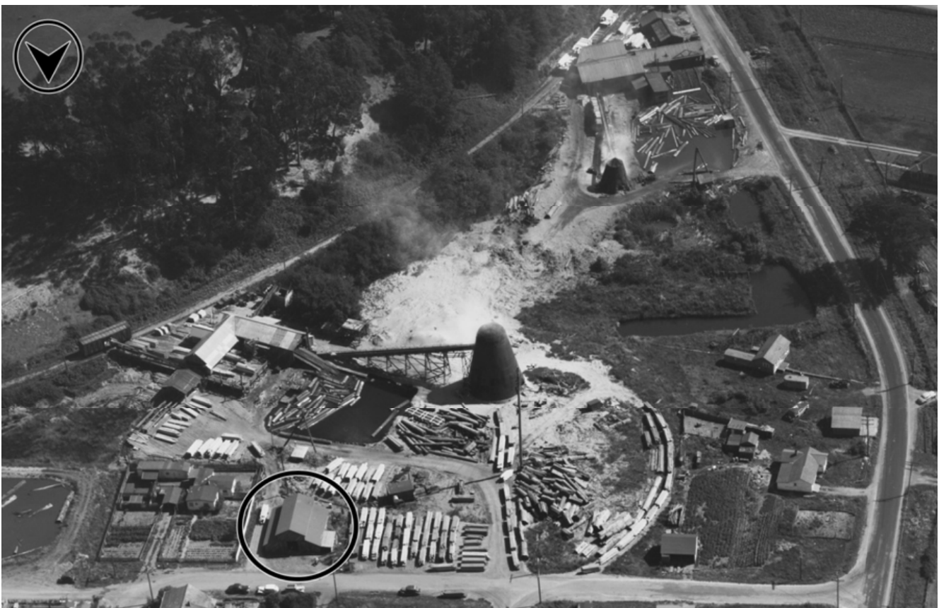
1947 aerial view of Speier's Mill B property, existing shop building circled, Alliance Road at right.
